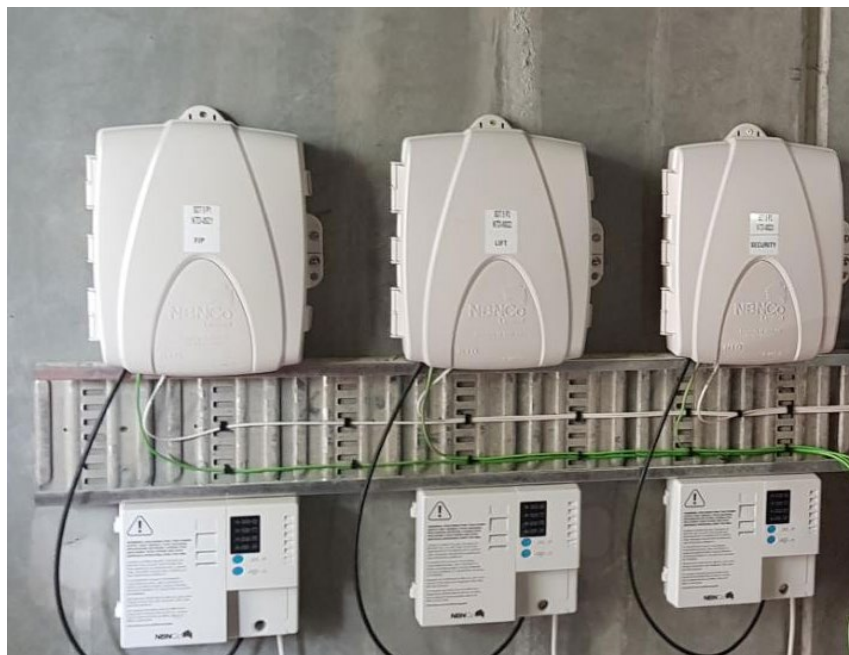
Figure 47. Centrally located Outdoor NTDs for essential services.
