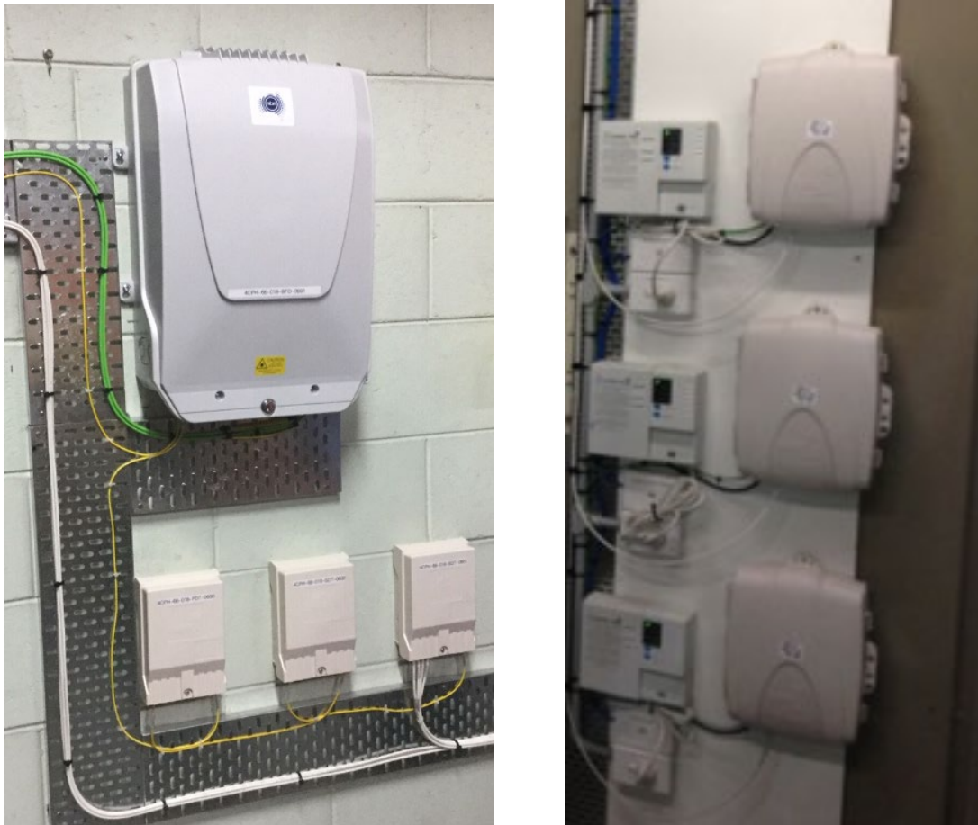
Figure 28. Example of typical communications room Budi and SDTs and BBU and Outdoor NTD
