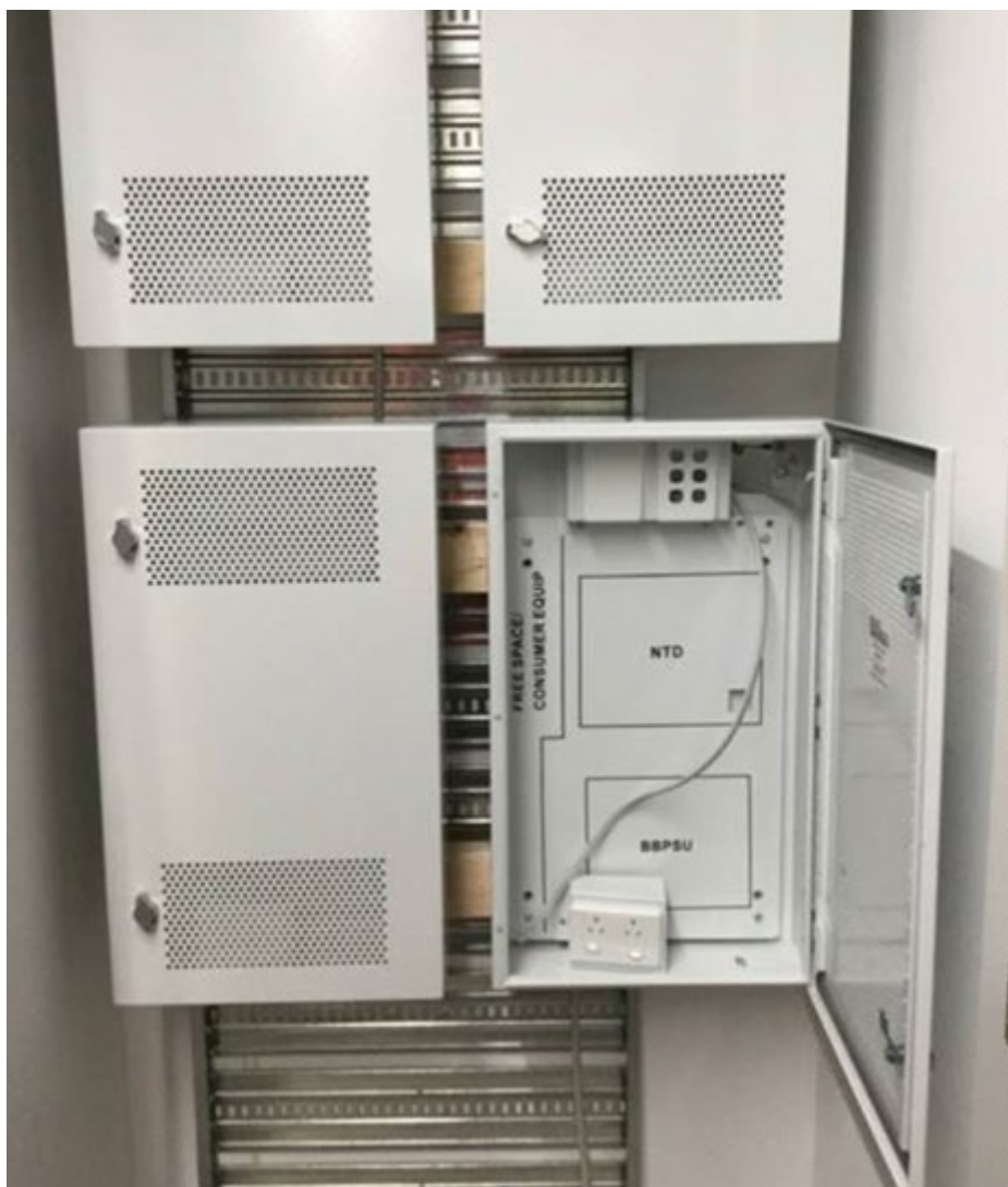
Figure 49. Centrally located NTDs with standard portrait layout within commercial developments
