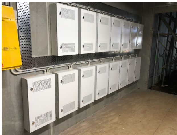
Figure 48. Centrally located NTDs for commercial developments.
